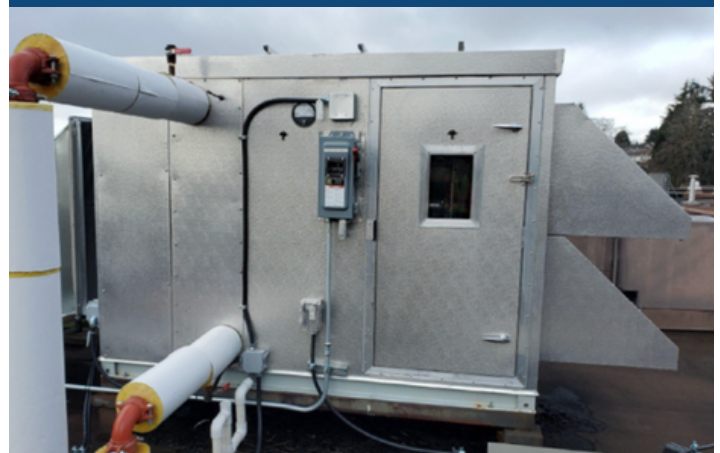
Image 2: Heat recovery coil into exhaust air stream (major waste heat source - after retrofit). Source: Ben Mills, Impact Engineering (2).
