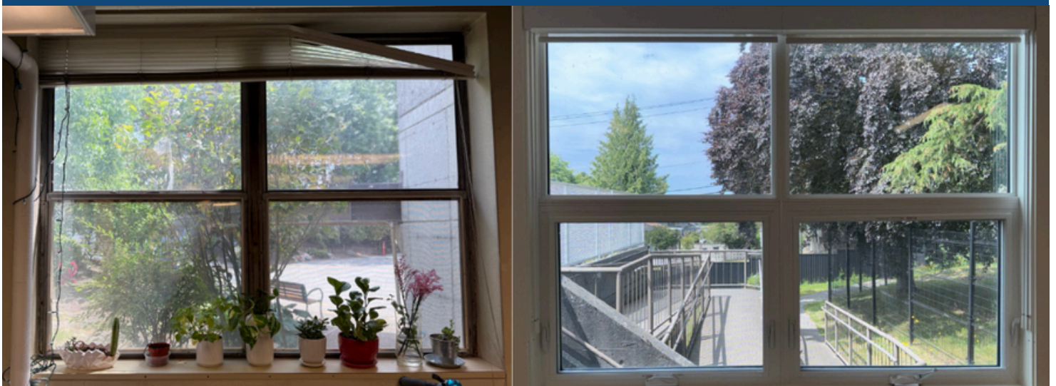
Image 7 (left): Original 1954 single-pane windows, before replacement. Image 8 (right): New silex 2100-series triple-glazed windows. Source: George Gemmel, Providence Health Care (2).
