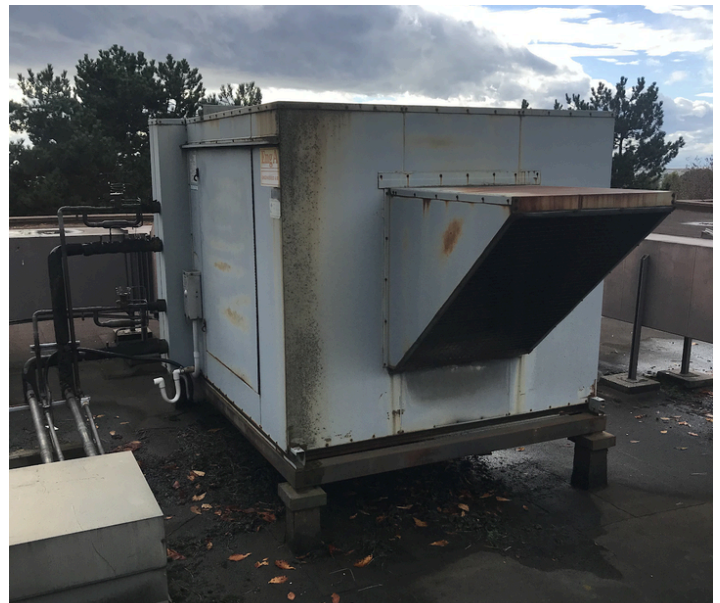
Image 1: HFH rooftop unit (before retrofit). Source: Ben Mills, Impact Engineering (2).
