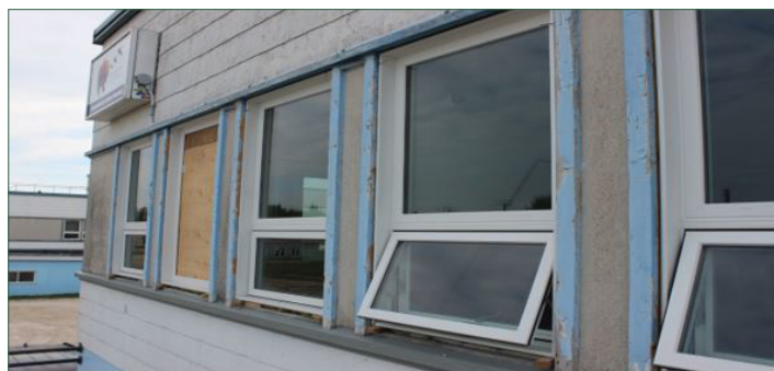
Replacement windows being installed at Weeneebayko General Hospital with some windows locations eliminated - awaiting filler panel installation, insulation, flashing, trim, and caulking.
