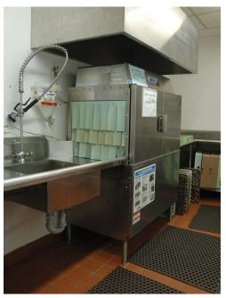
When a dishwasher uses less water, energy is also saved through a reduced need for water heating. ENERGY STAR qualified commercial dishwashers use approximately 25% less energy and water than standard models.
