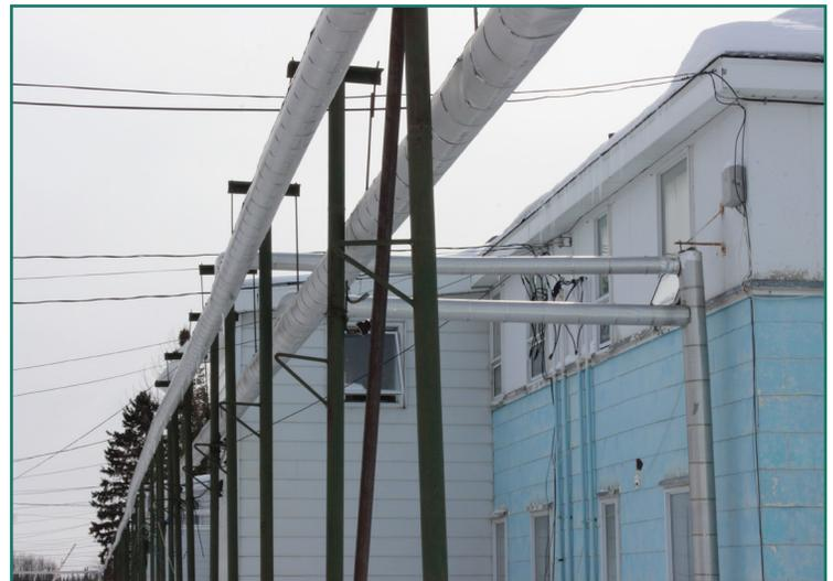
*Since repairing the condensate return line system at the Weeneebayko General Hospital in 2017, the results have been amazing! In place for over two years, there have been no incidents of freezing, splitting or rupture.*
